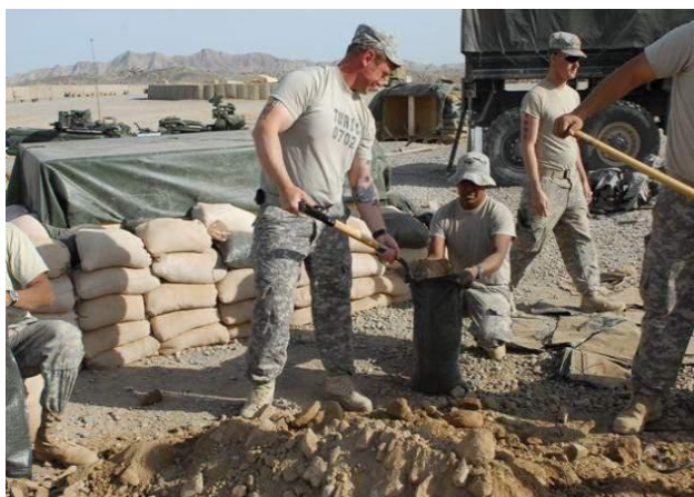
(SSG Turic, C Battery, 3-17 FA, helps his platoon fill sandbags for the 155mm ammunition bunker)
